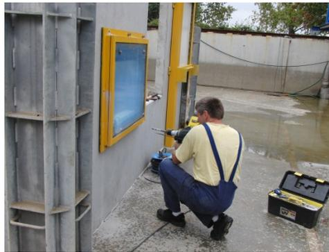
Fig. 6: Installation of the barriers
