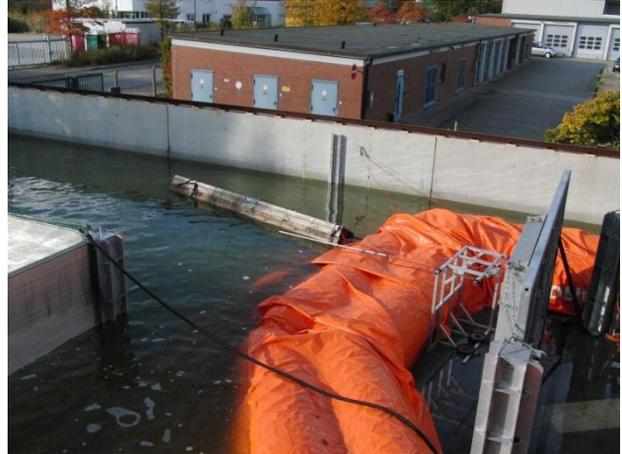
Figure 27: Mobildeich system – temporary perimeter flood barrier consisting of water-filled tubes
