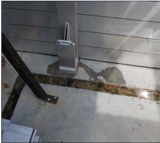
Fig. 2: Leakage at the supporting post<sup>36</sup>
