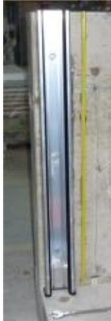
Installation of columns: connection to support with 3 anchor for each column
