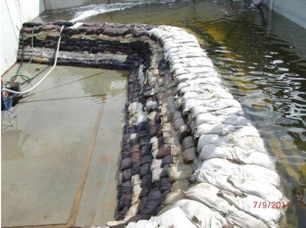
Figure 26: Sandbag system – temporary flood barrier
