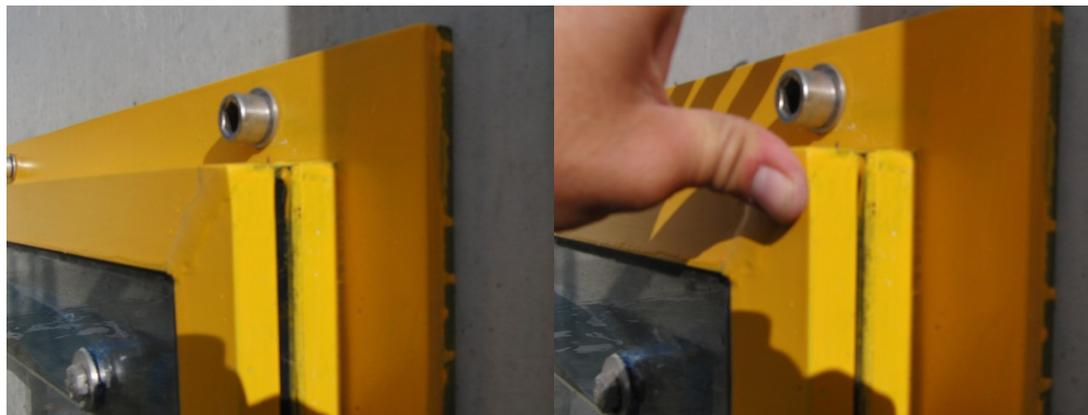
Fig. 7 (left) and Fig. 8 (right): The barrier for the basement window does not close properly
