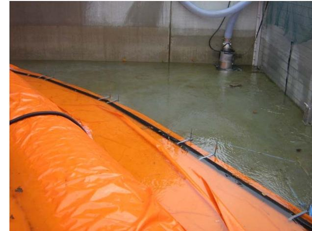
Fig. 5: Configuration of the Mobildeich using steel dowels
