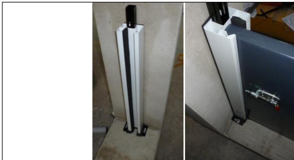
Installation of column with its steel frame and fixation with 2 anchors at the base of the steel frame, to create steel reinforced PVC column.
