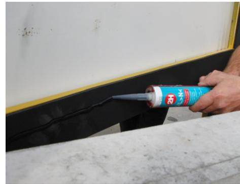
Fig. 7: Silicon spread over the gasket
