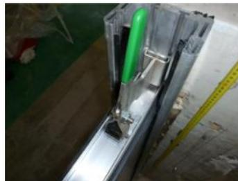
Installation of the vertical press (one for each column)
