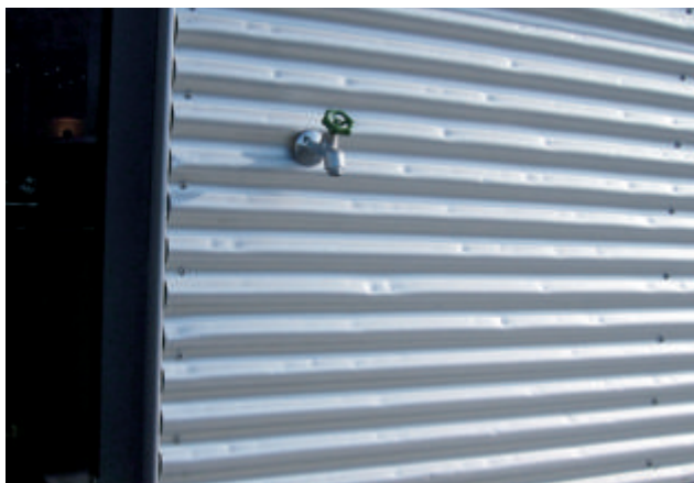
Figure 6.7: Tôle de façade, photo AVA.
